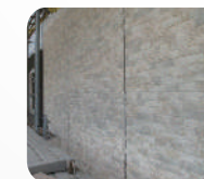
▼ Exterior-wall use Nano-coating
