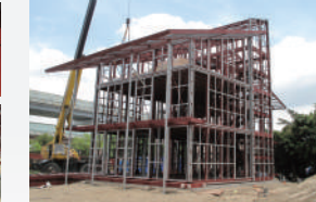
▲ Spending 3.5 days on the construction installation
