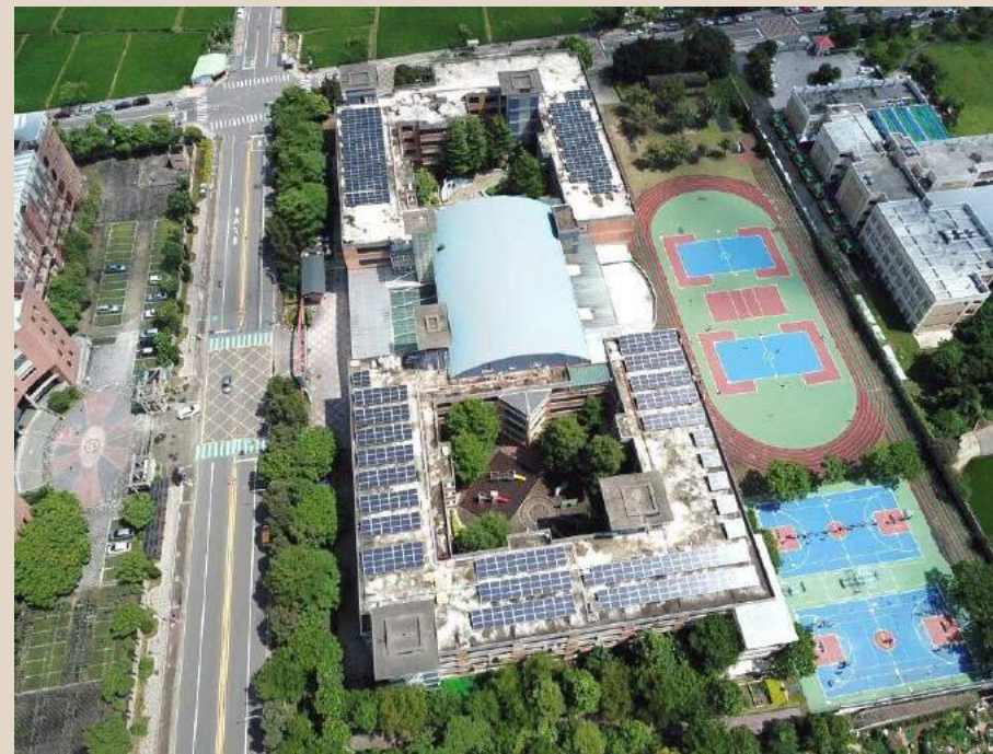
建德國小0.23MW
