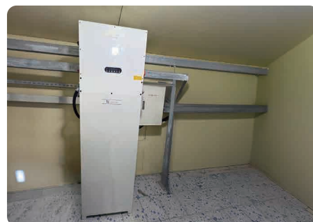
Energy Storage 11.5kW/19.8kWh
