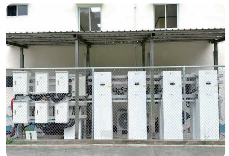
Energy Storage 103.5kW/178.2kWh
