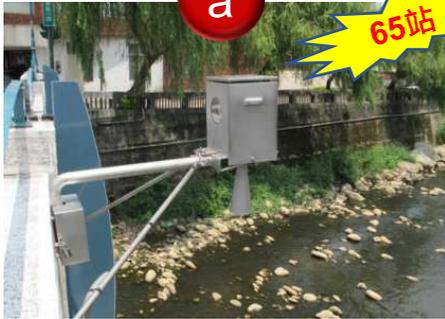
Drainage facilities control stations are set up near the important water gates for intelligent remote control.
