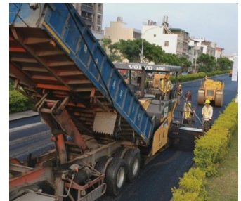
Pilot road with oxidized slag was paved on Fengde Road, Bade District
