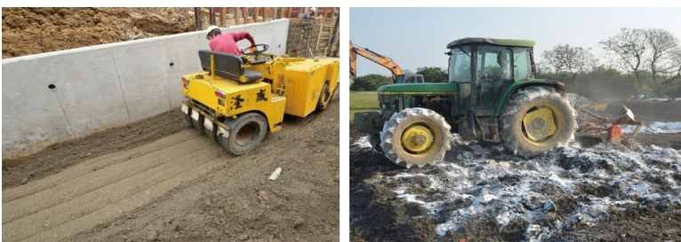
ICA were used for soil-strength mixing and backfilling in Fuyuan Park for rolling and pressing operations.(left)
