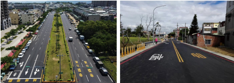
The trial road with oxidizing slag pavement completed on Fengde Road, Bade District. (left)
