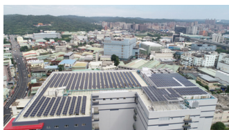
Installing Roof Photovoltaic Systems in Private Housing
