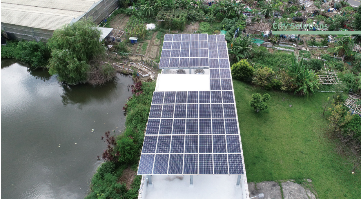
Solar photovoltaic system in a landfill.
